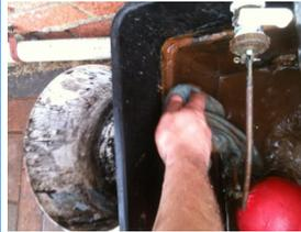
7. The Header tank, or F&E tank, (if present) is then cleaned until all sludge is removed.
