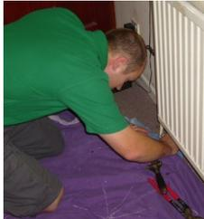
3. The machine is then switched on and all radiators are again checked to ensure that there is no weeping at the valves or elsewhere.
