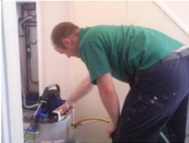
4. The dirty water is then dumped and the system is re-filled with clean water.
